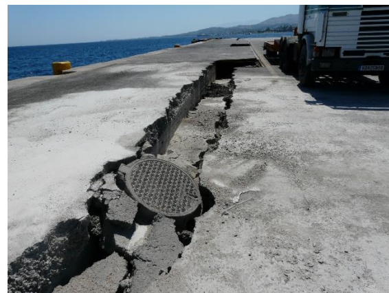
Figure 1. (upper left) Earthquake-induced ground failures at the cape Louros (photo taken by G. Papathanassiou on August 13, 2017), upper right) liquefaction manifestations at the area of marina that is used as a dry dock and for the maintenance and repairs of sailboats and yachts Louros (photo taken by G. Papathanassiou on August 13, 2017), lower left) lateral spreading phenomena induced damages to custom building (photo taken by G. Papathanassiou on August 14, 2017), lower right) failure at the new port of Kos (photo taken by G. Papathanassiou on August 14, 2017).
