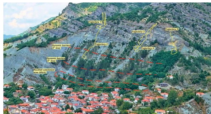
Figure 3. Recommended construction sites of dynamic rockfall barriers and ditches at the toe of the slope.
