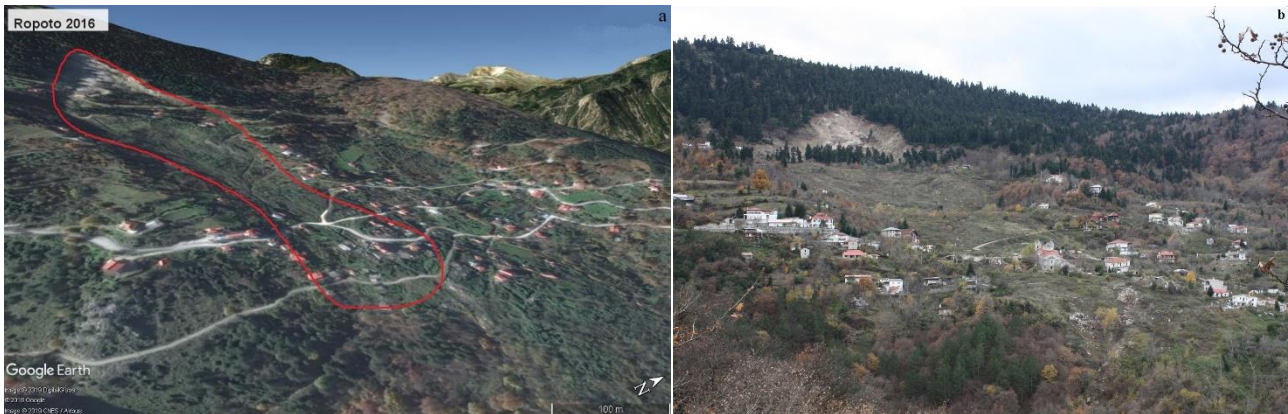
Figure 1: Aspect of Ropoto landslide: a) 2016-Google earth, b) 2018-Image.
